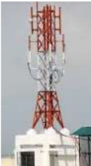
roof top tower.jpg 9K
